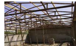
Construction of 4 secondary classrooms was sponsored by the Japanese Government
